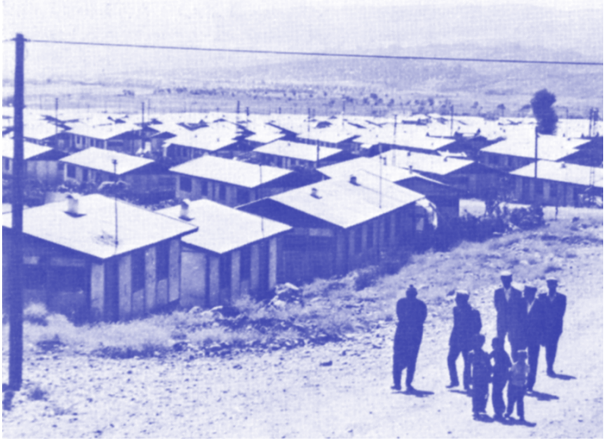
Prefabricated housing built by the Turkish Government at Lice following the earthquake of September 1975. Many families objected to the form and siting of the housing. These objections related to their lack of participation in what was provided, and the cultural and climatic unsuitability of the housing.
