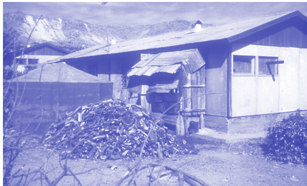
This picture illustrates three types of disaster assistance following the Lice earthquake in Turkey in 1975. On the right, a pre-fabricated house as provided by the Turkish government; on the left an emergency shelter made of polyurethane provided by OXFAM; and in the centre, an improvised addition to the house made by occupants. Many families objected to the form and siting of the housing. These objections related to their lack of participation in what was provided, and the cultural and climatic unsuitability of the housing. OXFAM used their polyurethane house for the first and only time. Four hundred and sixty-three units were produced.
