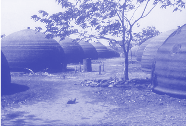
Adjacent to the El Coyotepe campsite in Masaya, Nicaragua, following the 1972 earthquake the West German Red Cross donated 500 polyurethane igloos. Although such units only take two hours to fabricate, it took 148 days for the first igloo to be occupied due to logistical problems as well as difficulty in obtaining a site with approval to build. Approximately 30 per cent of the igloos were occupied despite the fact that there were no rent charges.
