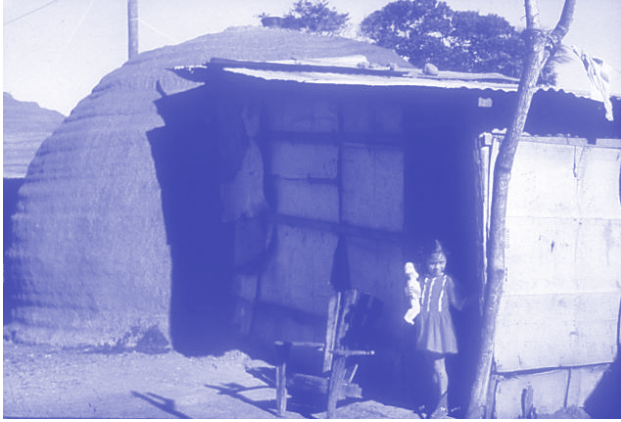
El Coyotepe, Masaya, Nicaragua. Fifteen months after the igloos had been built, families had already made extensive additions/modifications. Note the rectangular profile of the additions, to suit local building traditions, in lieu of the alien circular form. Since the igloos could easily be cut, this proved very easy for such additions to be made.
