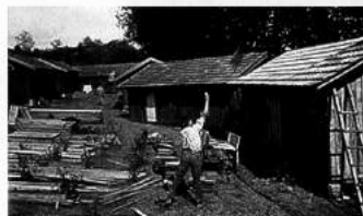
1917 Demountable Wooden House France (various locations) American Friends Service Committee Built by volunteers to house World War I refugees, each "demountable" wooden house consisted of two rooms. American Friends Service Committee
