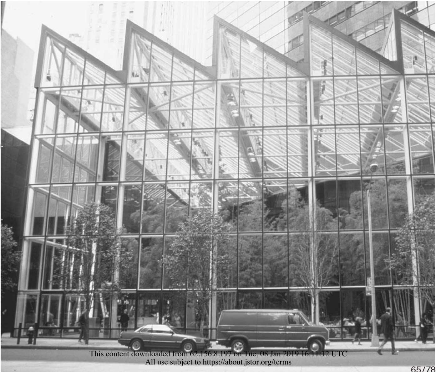
Figure 4.4. Exterior of atrium, 2001.
