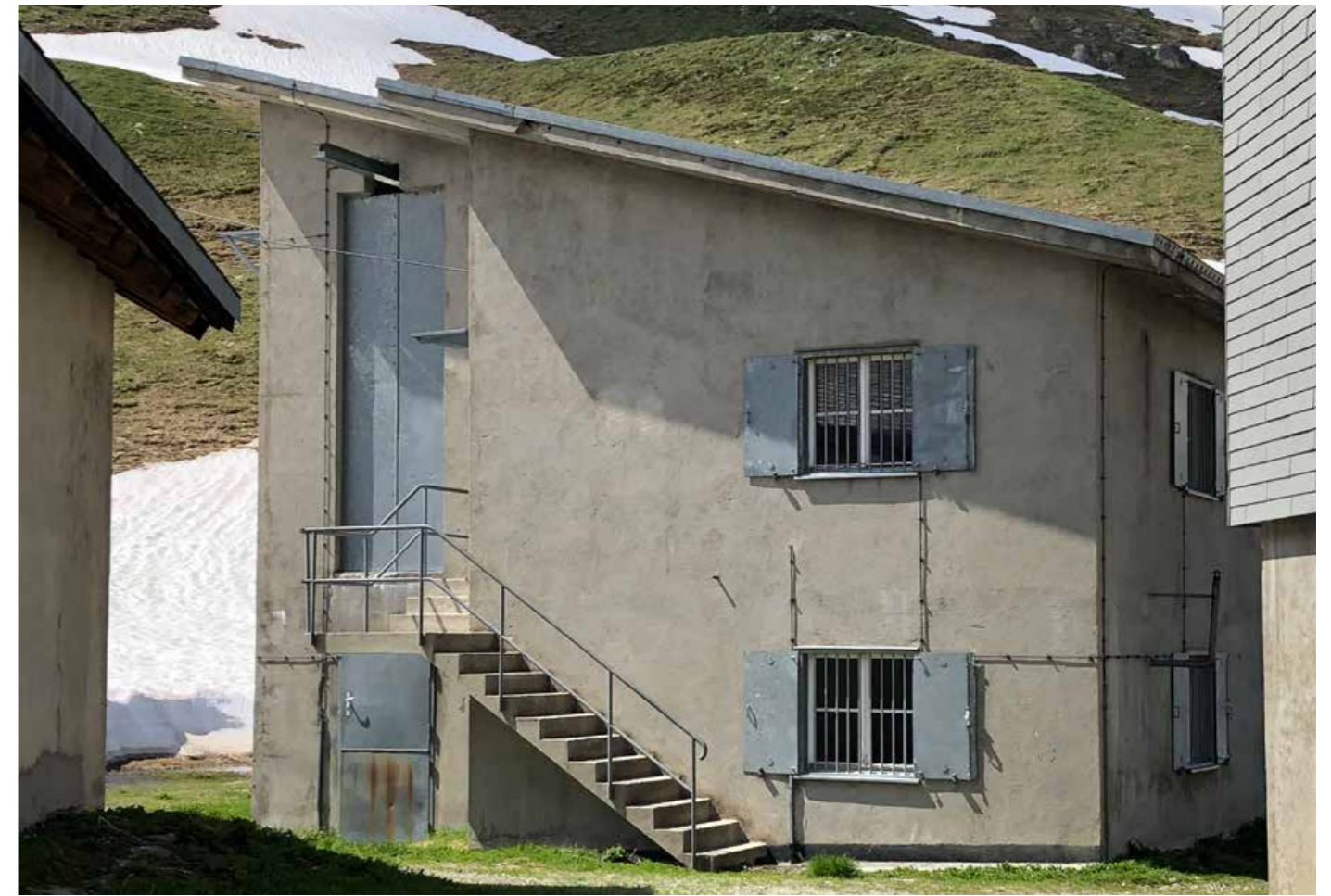
Military cableway which connect the camp to the Furkahörn, 2019
