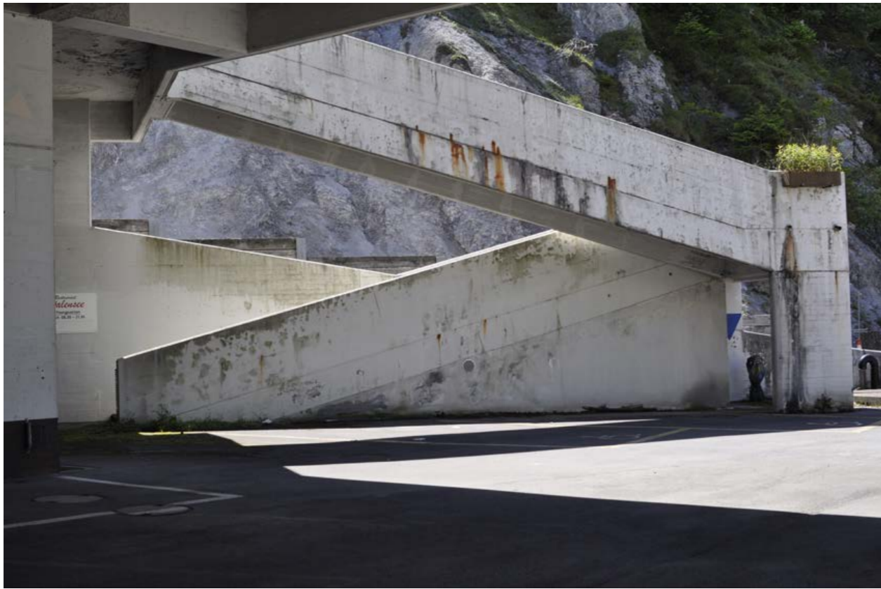
Staircase leading to the restaurant at the 2nd floor, 2017
