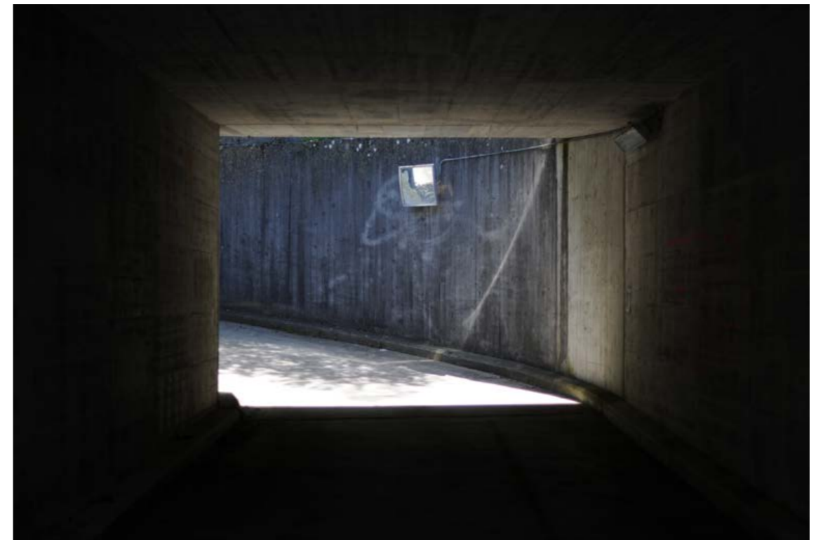
Underpass of the motorway A3, 2017
