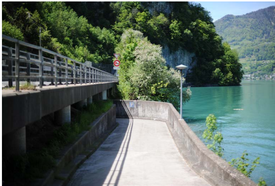
Way to underpass, 2017
