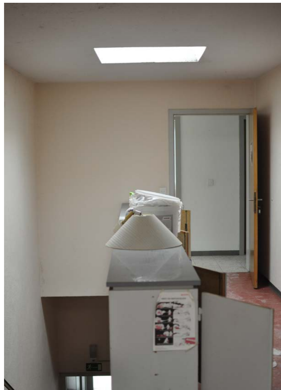
Third floor, corridor and staircase, 2017
