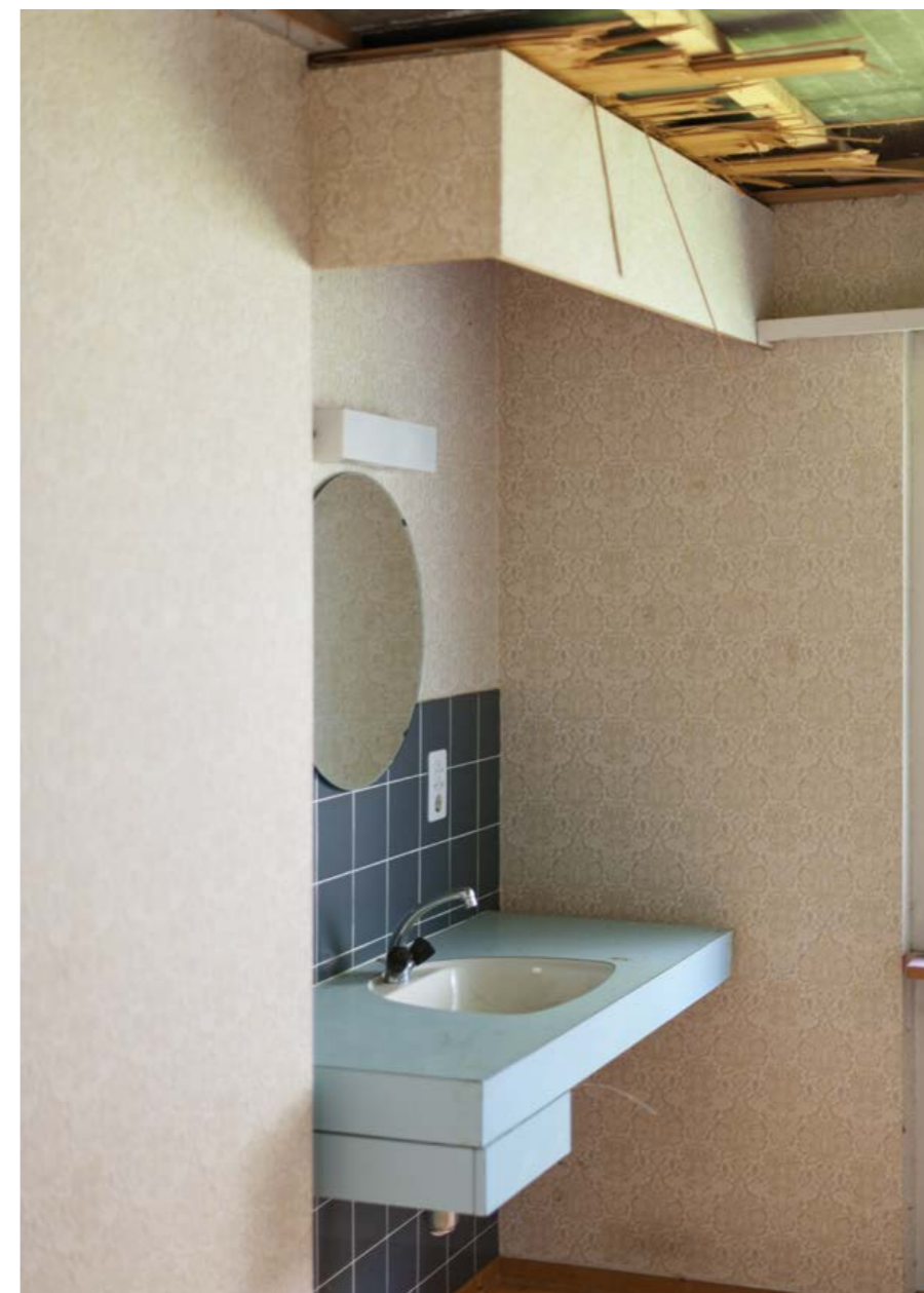
Third floor, bathroom, 2017
